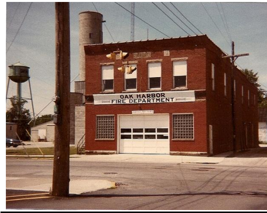
240 West Water Street – Community Hall 2 nd Floor
